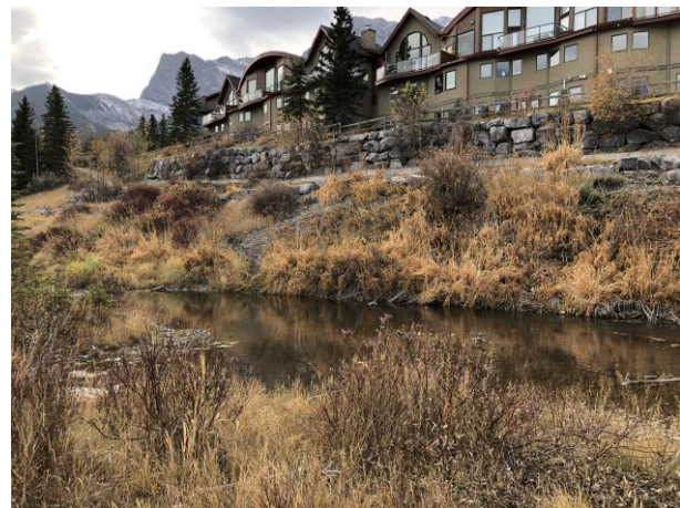
Figure 5.3 Upper Pathway Retaining Wall
