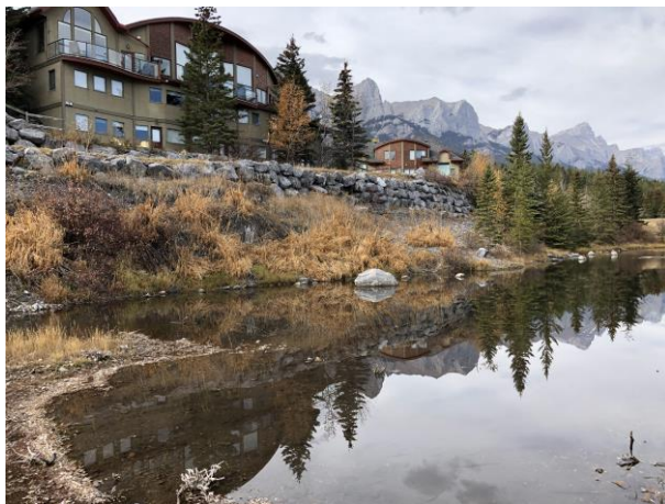
Figure 5.2 Creek Escarpment Retaining Wall
