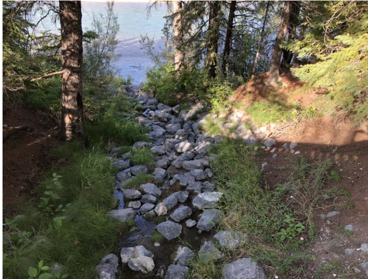
Figure 5.9 Homesteads Stormwater Outfall Channel
