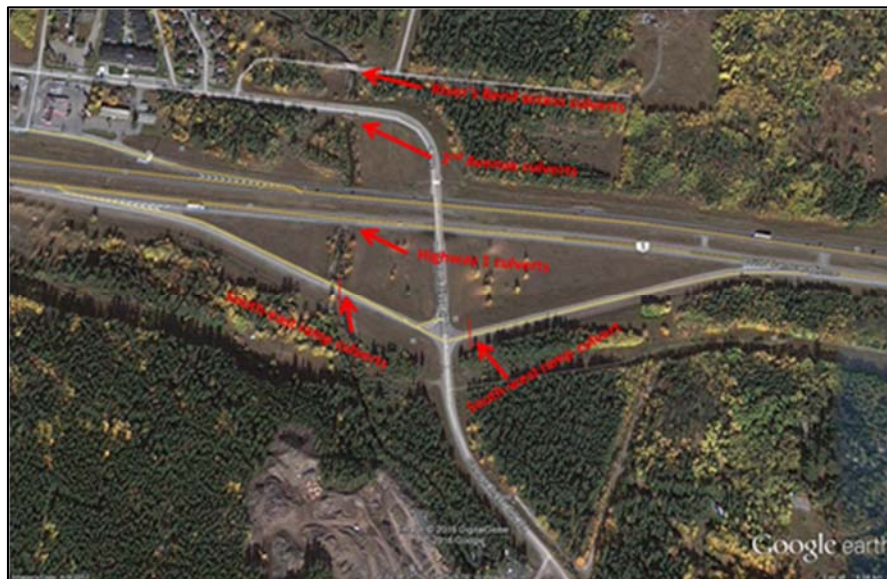
Figure 2-1. Location of blocked culverts considered in the Pigeon Creek hazard modelling (provided by Canmore, March 17, 2016). The south-west and south-east ramp culverts are mislabelled in this figure received from Canmore. At the time of writing, Canmore has indicated this is not anticipated to change the modelling scenarios.
