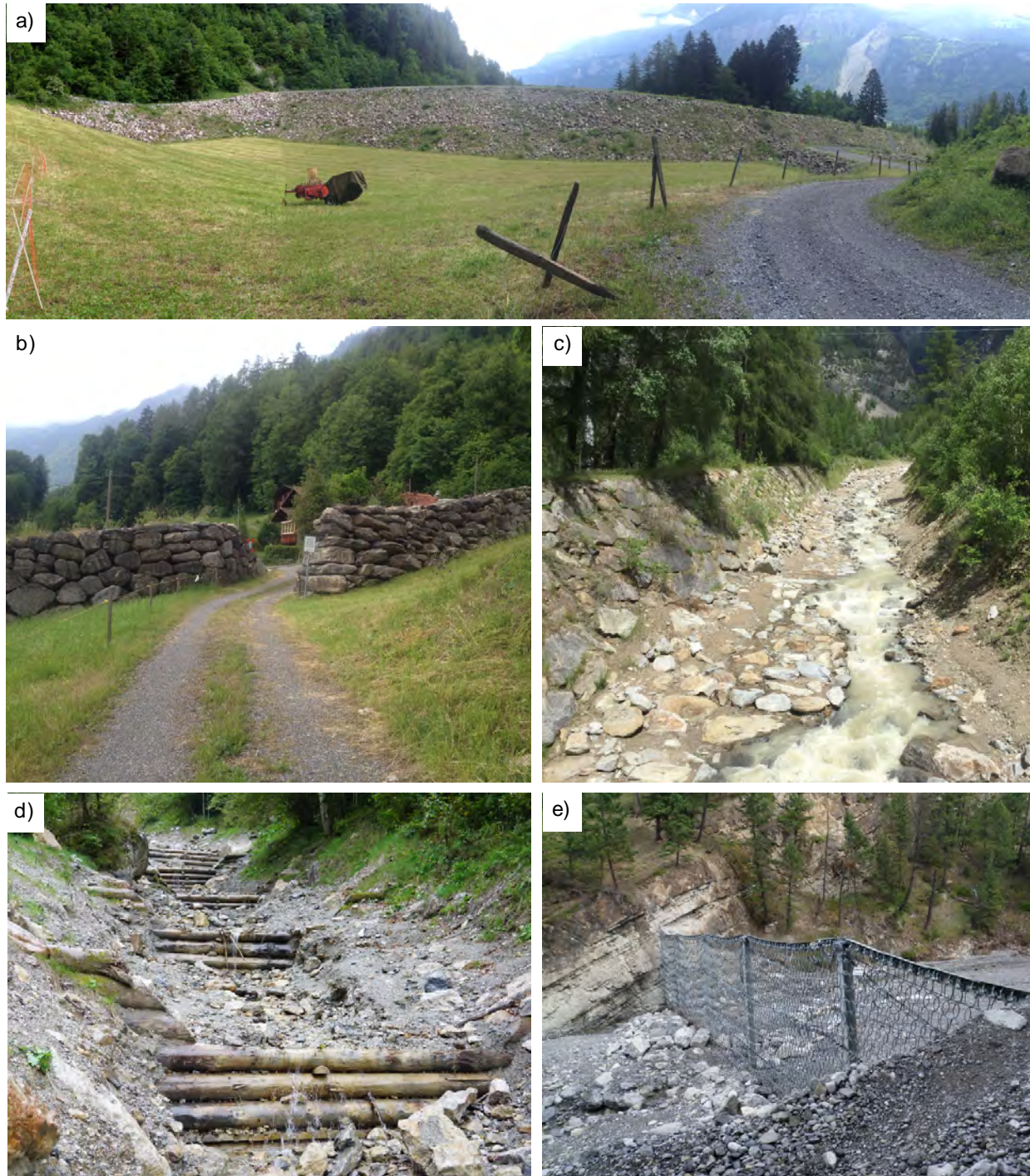
Figure 3-9. Examples mitigation structures: (a) earth-fill retention berm, Glyssibach, Brienz, Switzerland; (b) stone diversion berm, Trachtbach, Brienz, Switzerland; (c) conveyance channel with earthfill berms, Rennebach, Austria; (d) log crib check dams, Gesäuse, Austria; and (e) flexible debris net, Cougar Creek, Canmore, Alberta. Photograph (d) by M. Jakob, other photographs by E. Moase.
