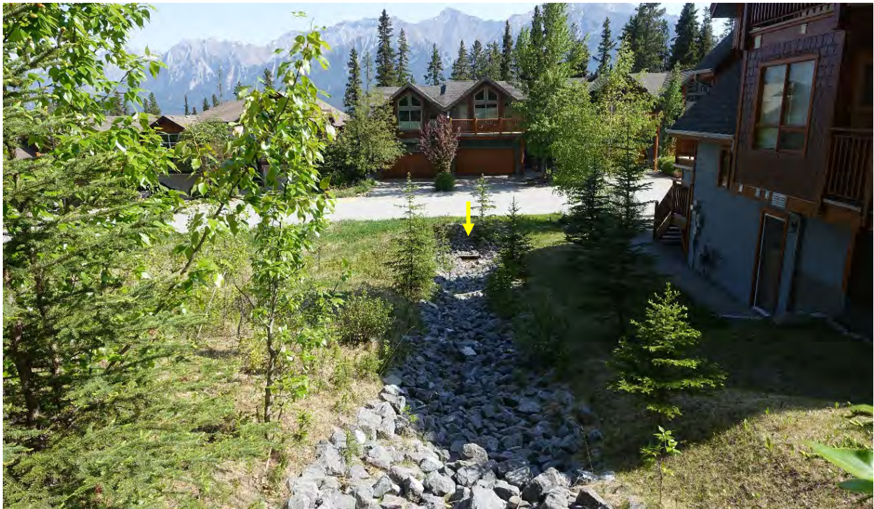
Figure 2-10. Looking downstream along the western Z Creek riprapped channel. Yellow arrow points to storm drain inlet at the far end. BGC photo, June 7, 2018.
