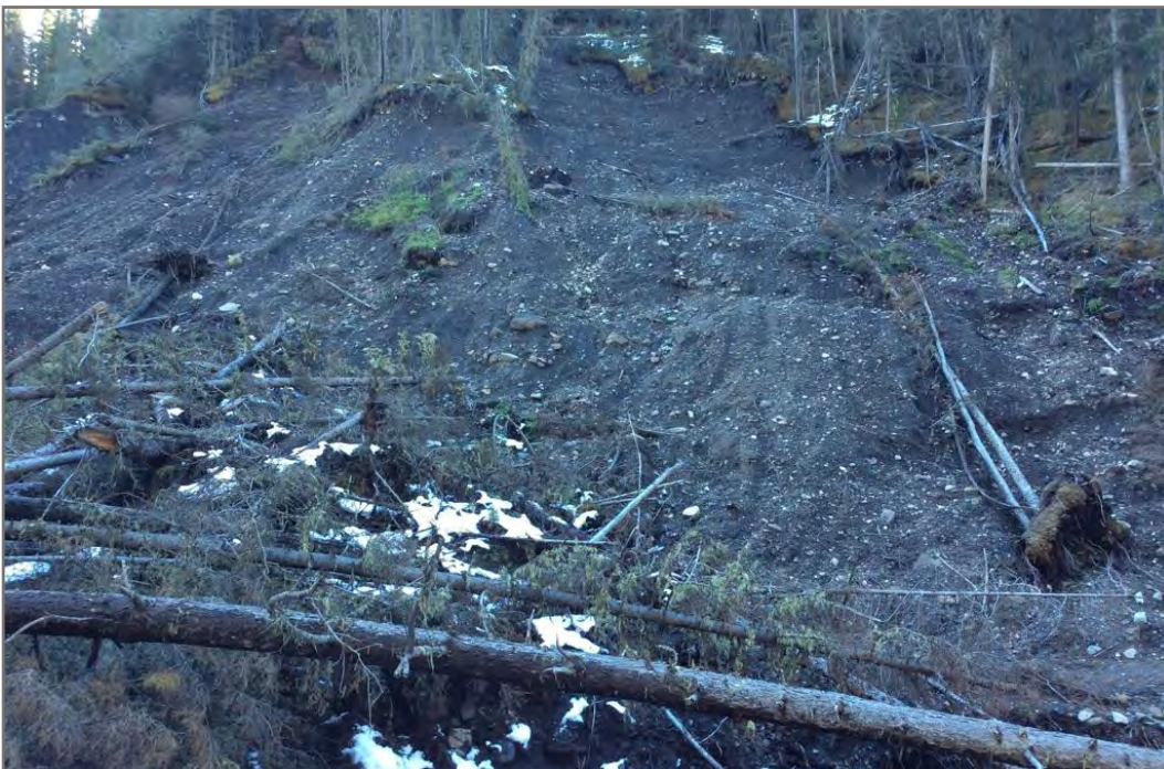
Photo 179(1): Failed slope in creek.
