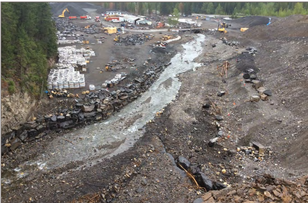
Photo 43(1): New position of Pigeon Creek in Thunderstone Quarry, near apex waterfall, looking north. Note limestone block riprap placed on west bank by Thunderstone Quarry operator.
