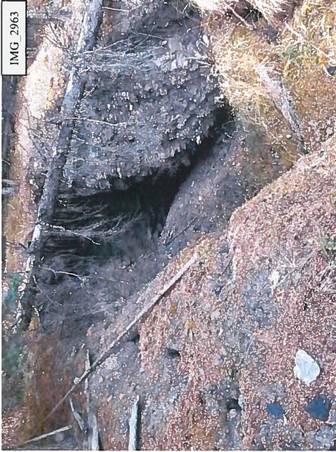
Photograph 5: Stewart Creek Golf Course Collapsed Portal Entrance Area (R19)
