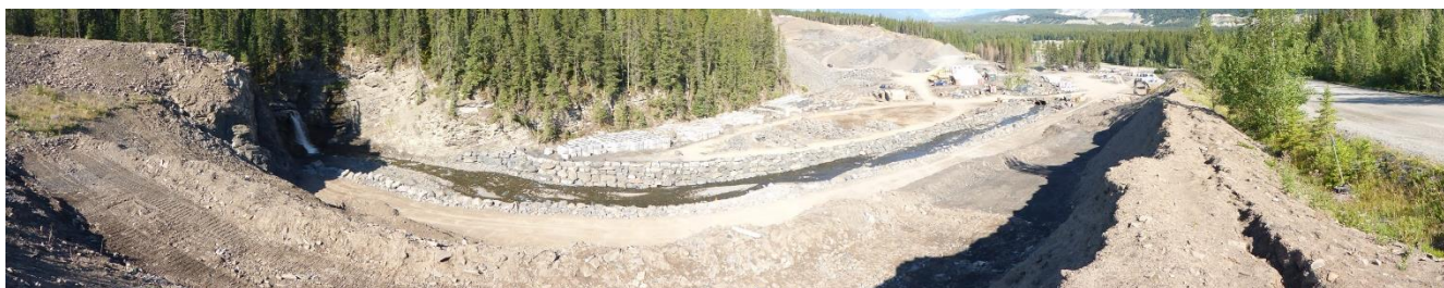
FIGURE 2: VIEWING NORTH, PIGEON CREEK DOWNSTREAM OF LOWER SPRAY FALL, FLOWING THROUGH THUNDERSTONE QUARRIES
