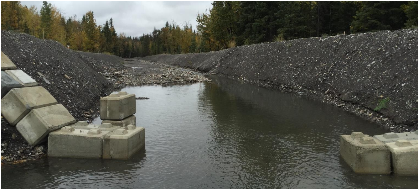
FIGURE 5: STATE OF CHANNEL CONSTRUCTION WORKS IN SEPTEMBER 2016 DOWNSTREAM OF RIVERSBEND ACCESS
