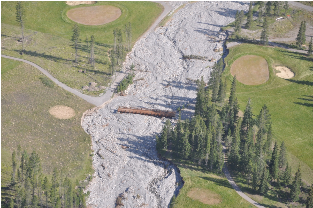
Figure 3-5. Aerial view of Three Sisters Creek looking downstream. The Upper Bridge was outflanked on both banks during the June 2013 debris flood. BGC photograph of July 23, 2013.
