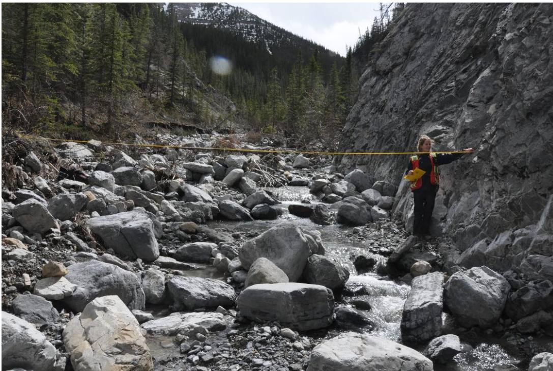
Figure B-2. Upstream view of Three Sisters Creek high water mark at WP3. BGC photograph of May 29, 2014.
