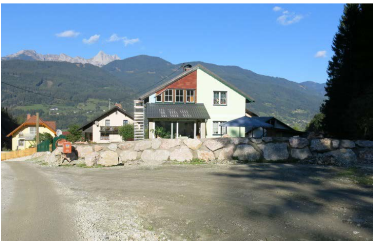
Figure EDCG HLC 9.5: Example of Raised Lot Grading with Stone Pitched Retaining Wall
