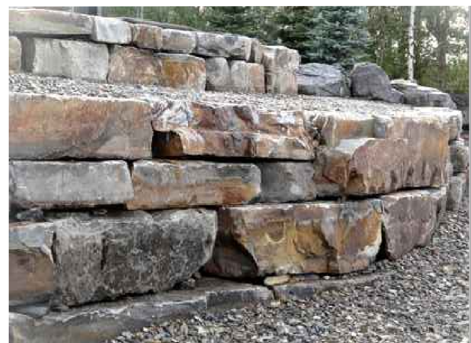
2 BOULDER RETAINING WALL - PRECEDENT IMAGE SCALE: NTS
