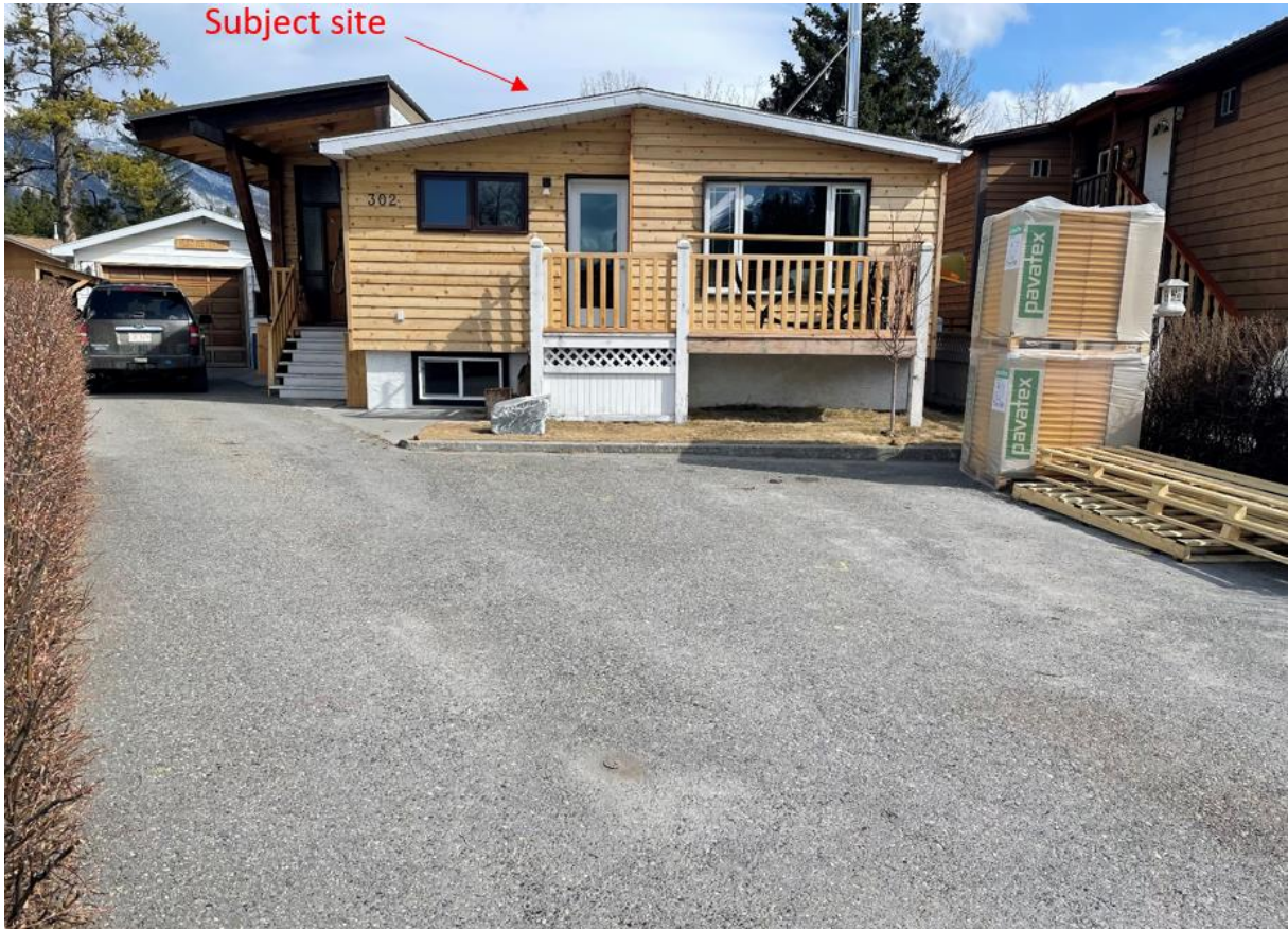
Close-up view at front of property
