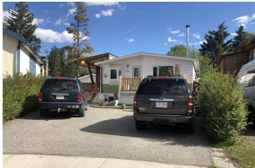
EXISTING FRONT FACADE
