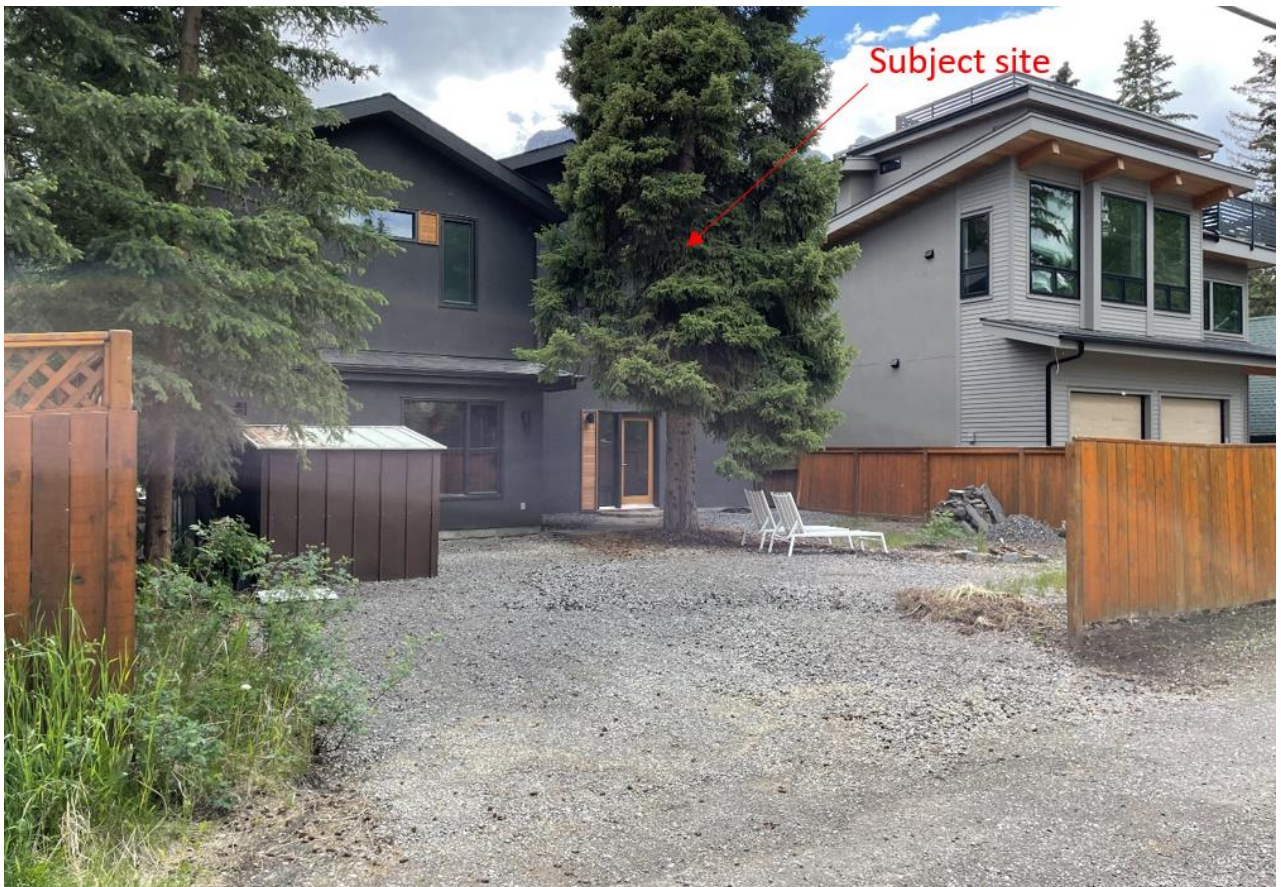
Looking south from the lane
