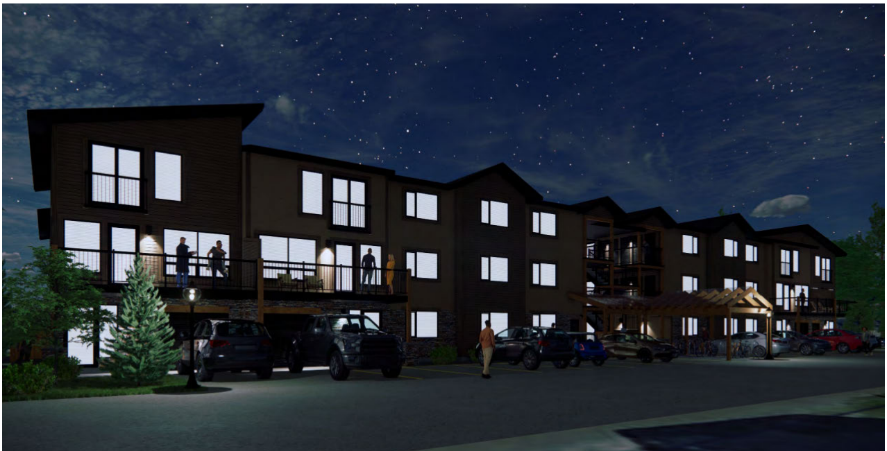
Rear Lane Fronting Buildings Exterior Lighting
