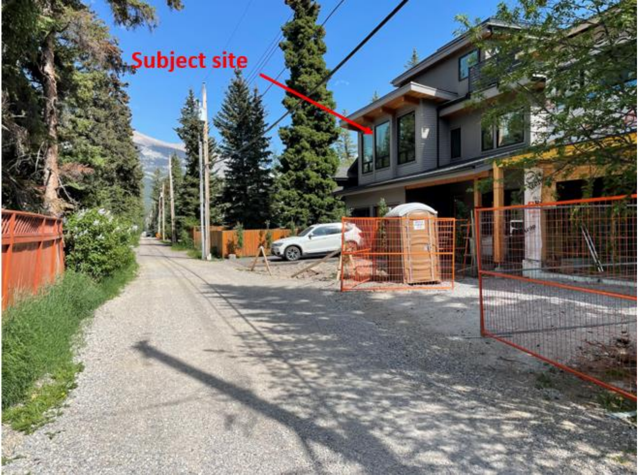
Looking east from lane
