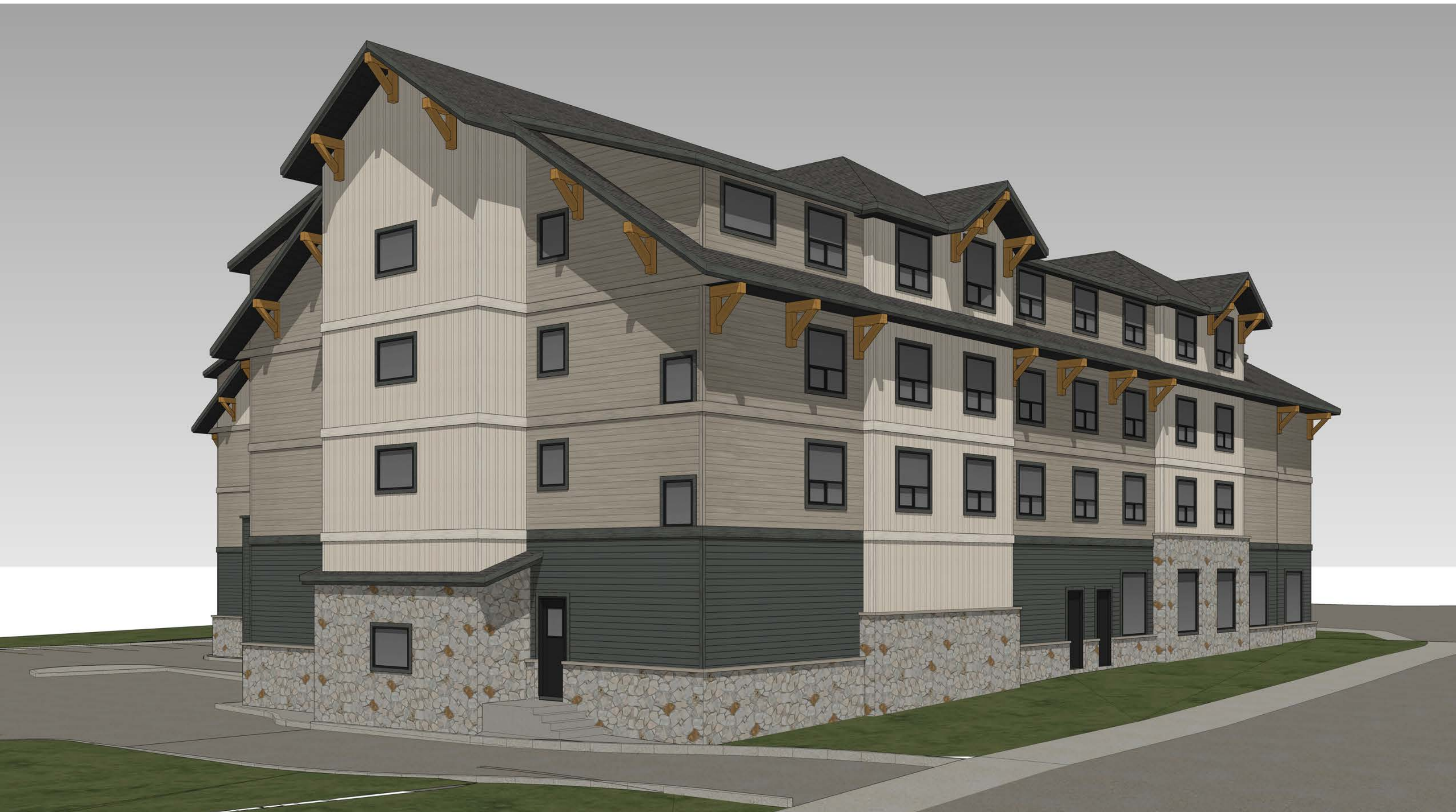
View of building looking East
