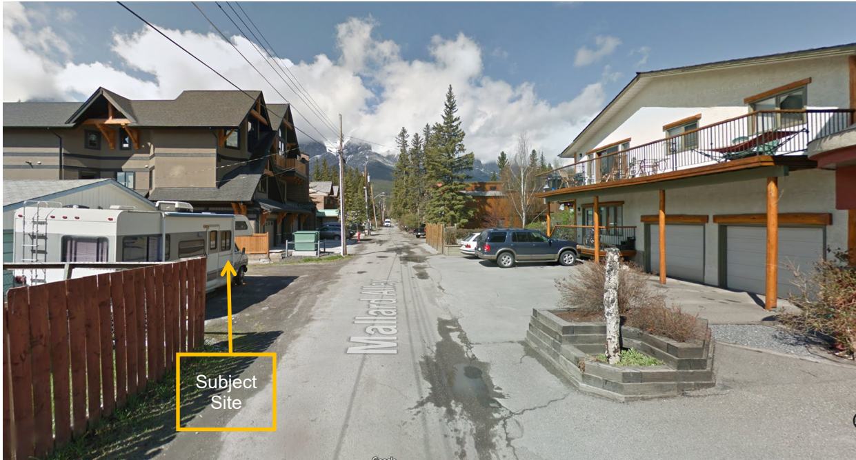
Street view looking West along Mallard Alley
