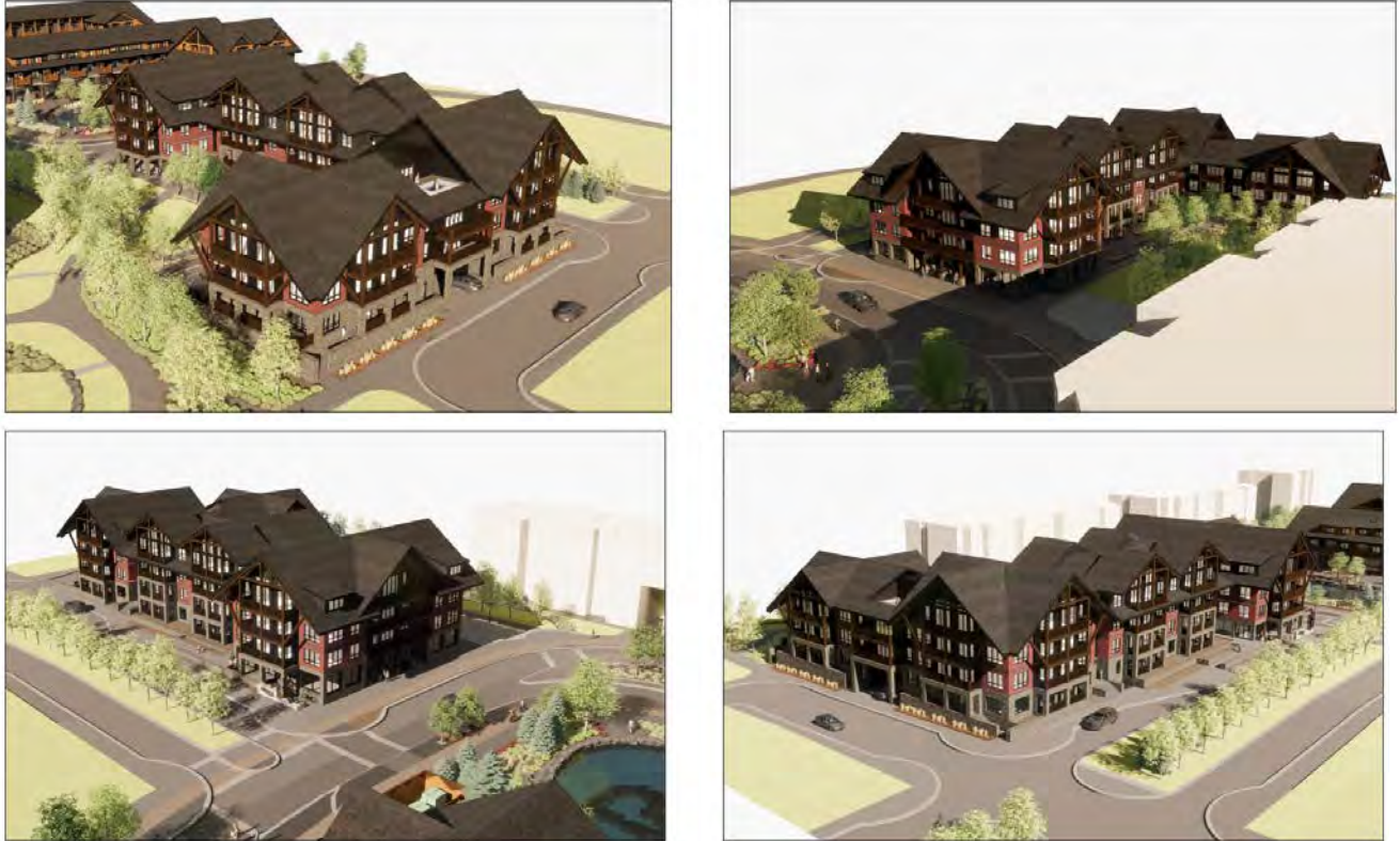
Figure 4 – Renderings of project (clockwise from top left: looking north-east, looking south-east, looking south-west, and north-west)
