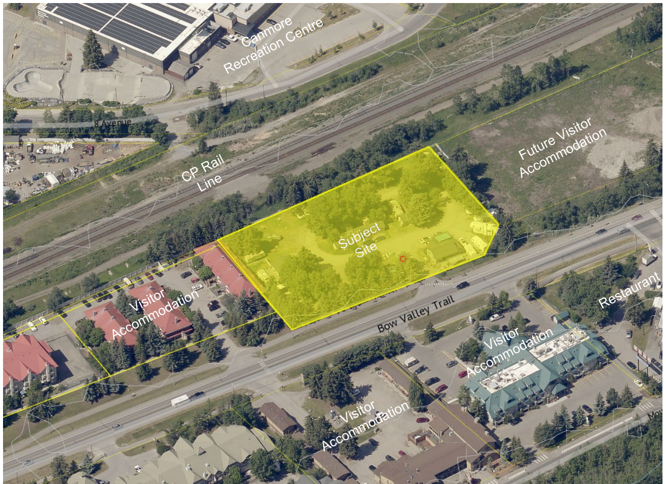
Figure 1: Overview of Site and Adjacent Uses (looking Northwest)
