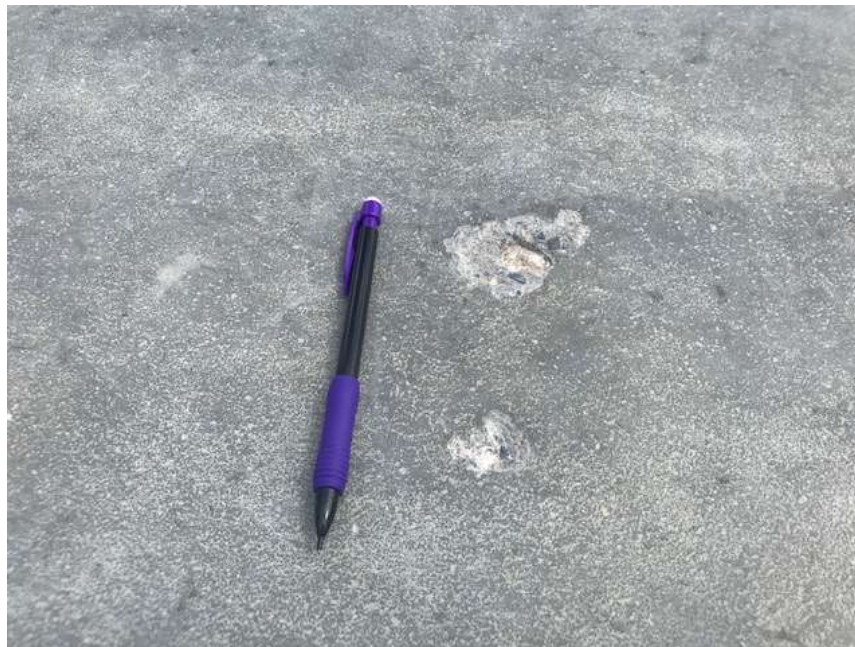
Concrete chips to grind / fill.
