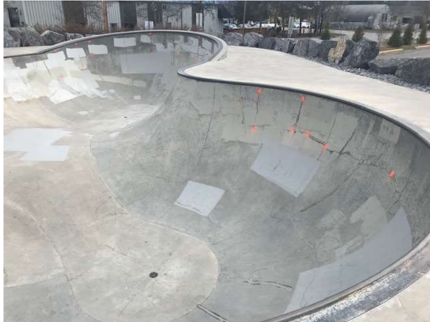
Cracks to grind and fill on ramp
