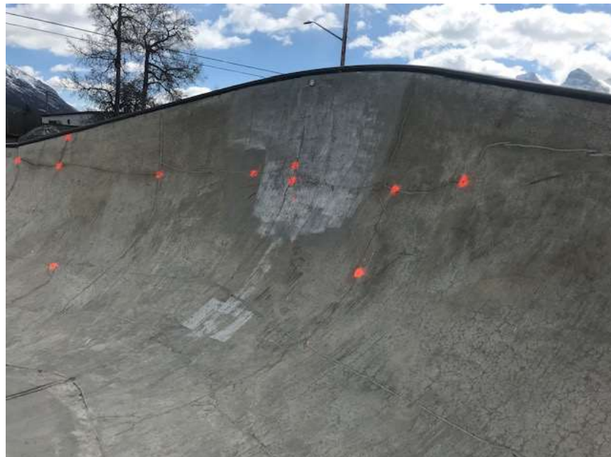
Cracks to grind and fill on ramp
