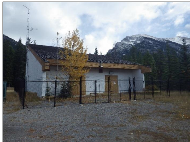
Town of Canmore Benchlands Pumphouse 4 with Combustible Wood-Shake Roof
