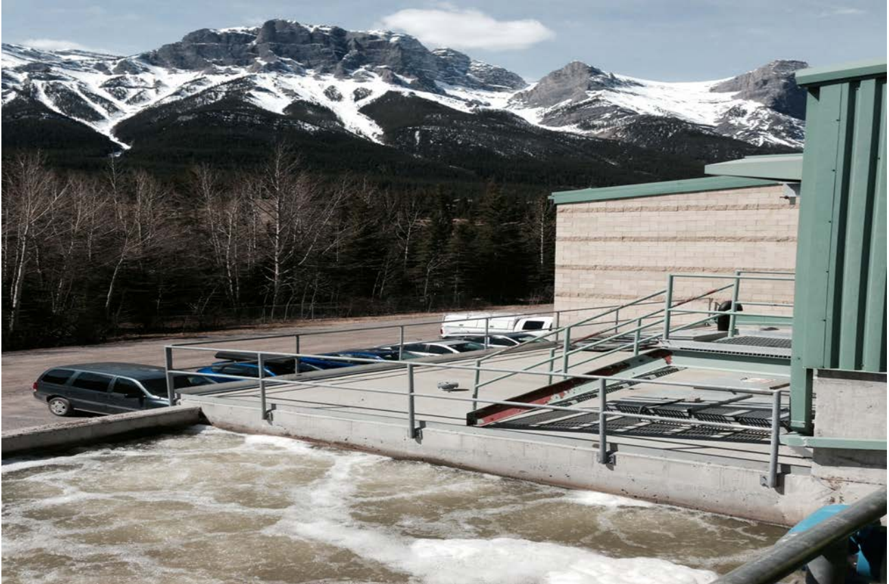
Figure 9: Wastewater Treatment Plant
