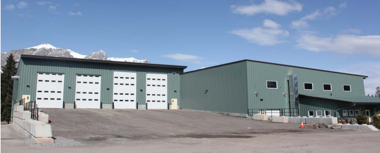
Figure 5: Materials Recycling Facility
