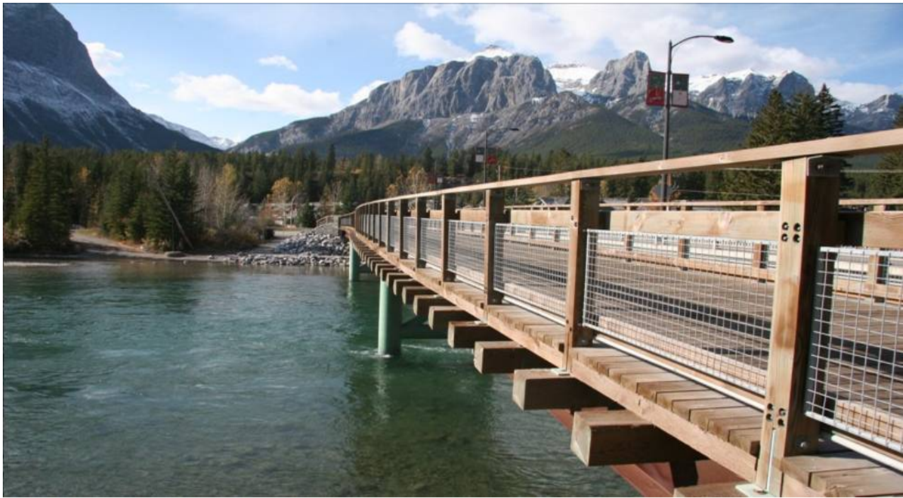
Figure 6: Bow River Bridge
