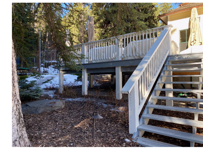
4. LOOKING AT EAST SIDE OF EXISTING DECK
