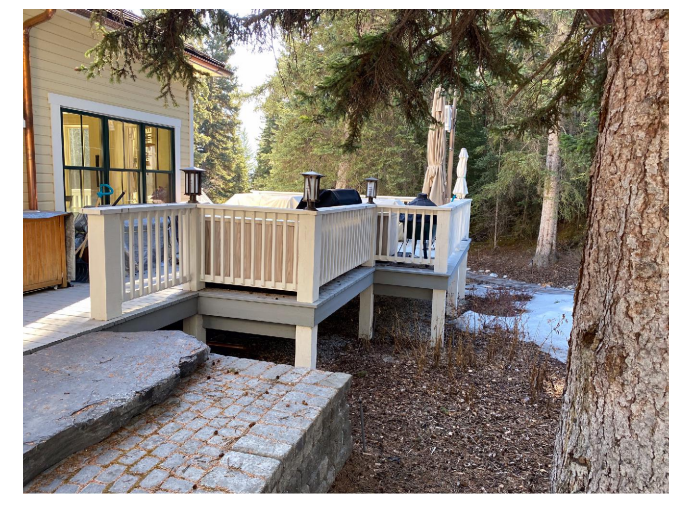
3. LOOKING AT EXISTING DECK FROM DRIVEWAY
