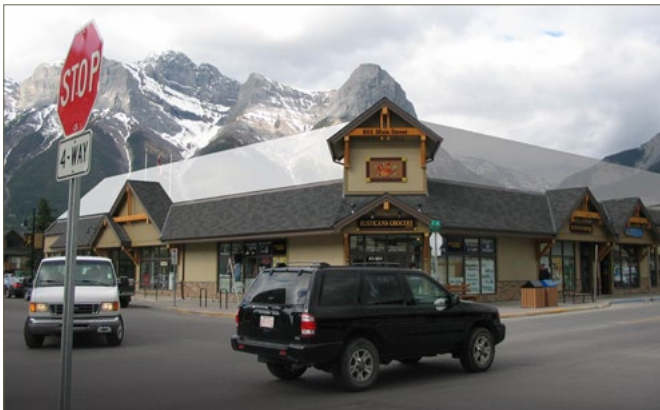
c) Main Street & 7th Avenue looking South-West
