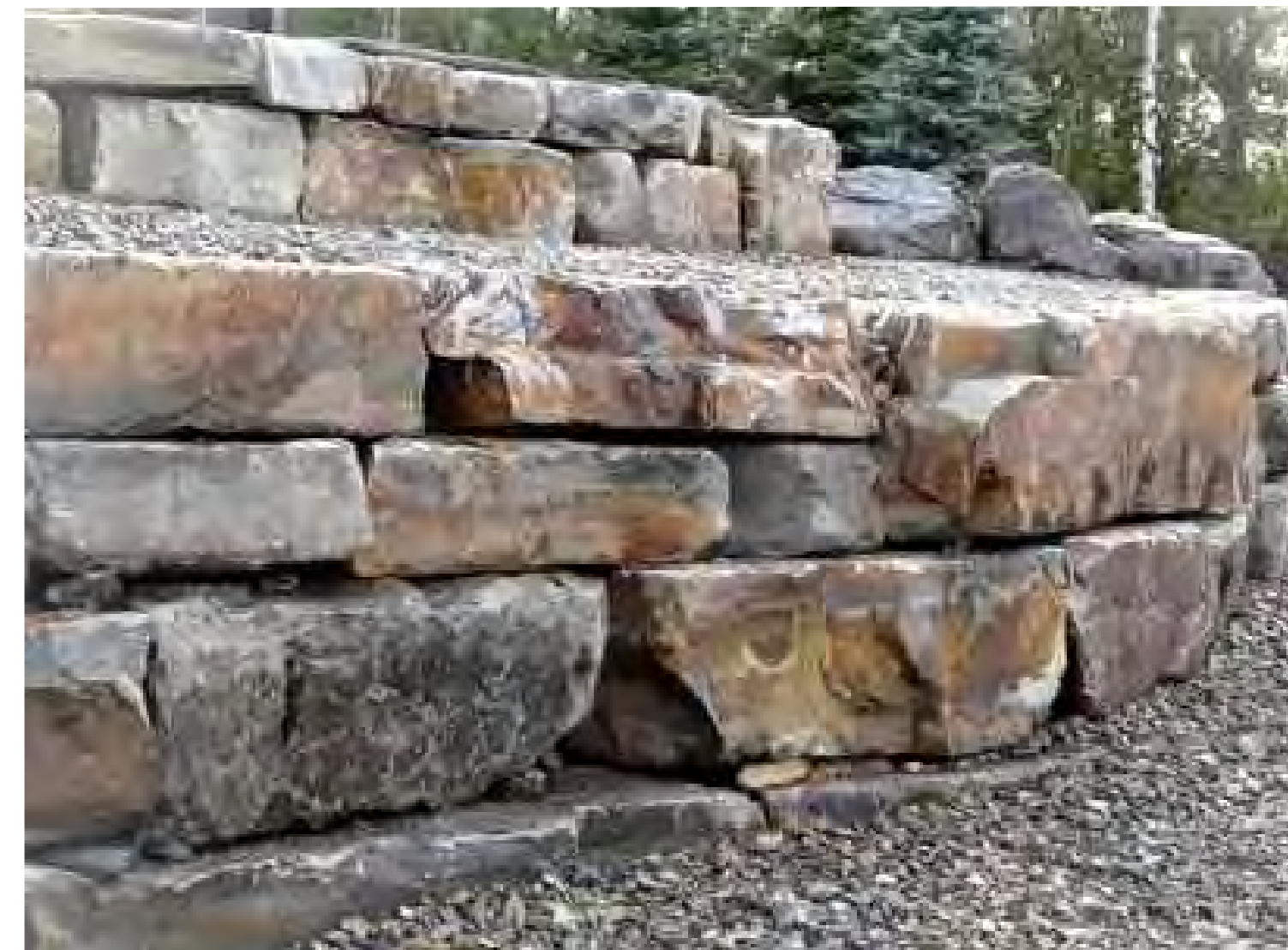
2 BOULDER RETAINING WALL - PRECEDENT IMAGE SCALE: NTS
