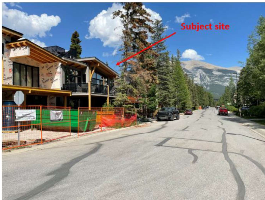
Looking east on 1 st Street
