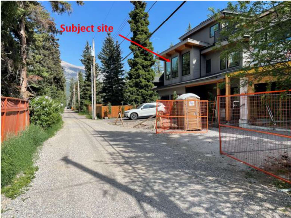
Looking east from lane
