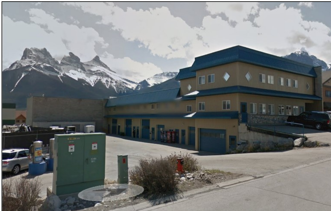
Photo of lower level units of Subject Site
