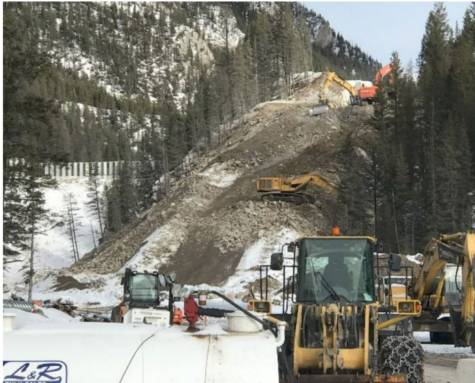
Spillway Chute, January, 2024 – Blast 1 Complete, Material Handling Underway
