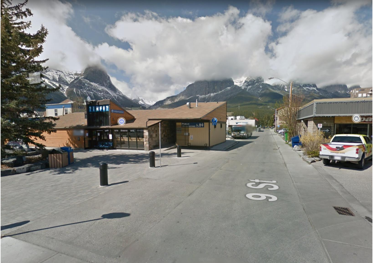
Figure 20: Front View of 9th Street Terminal (Source: Google Maps)
