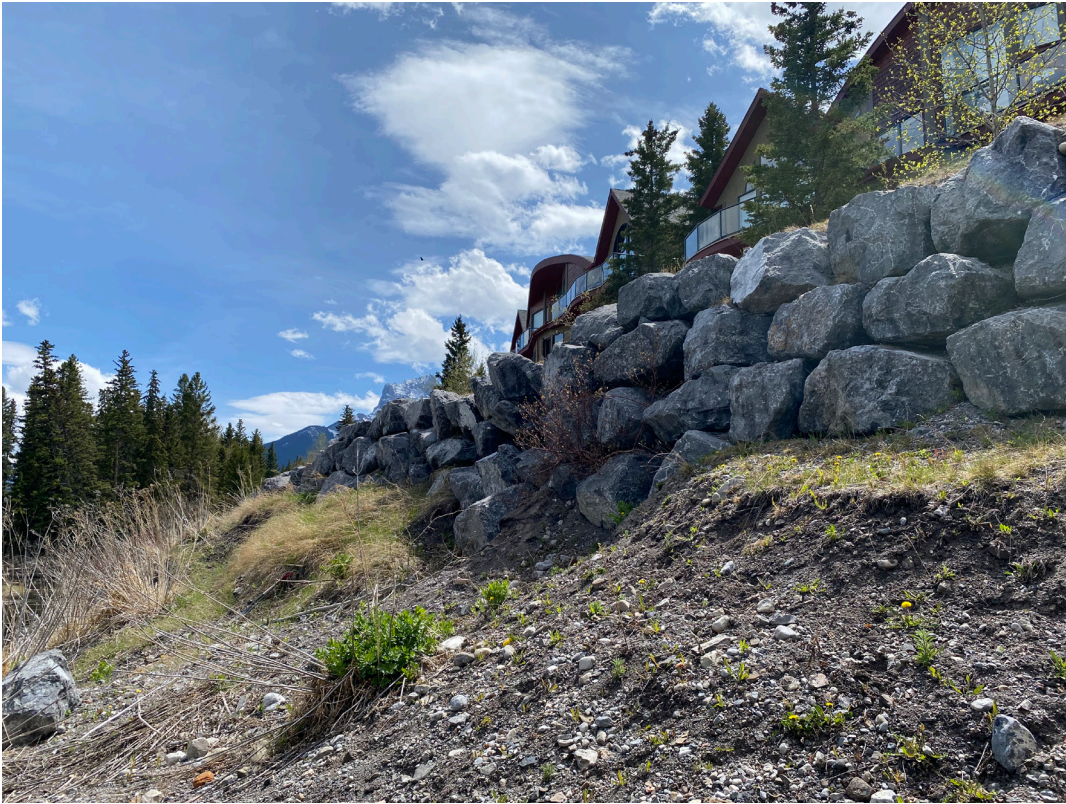
Photograph 1 Base of retaining wall facing East
