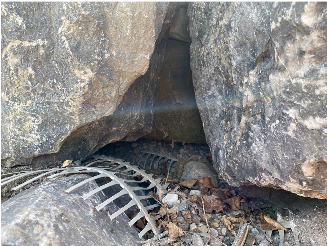
Photograph 4 Close up of the retaining wall
