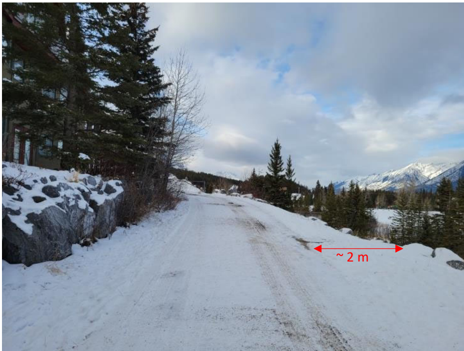
Photo 9: Location of wall relative to overlying pathway and upper retaining wall.
