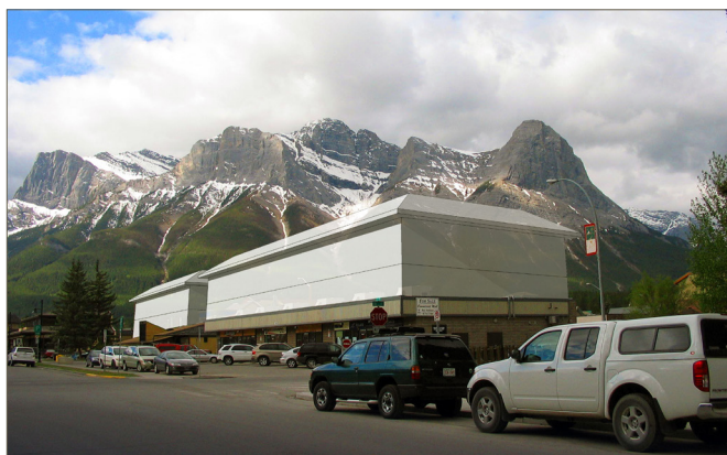
e) 10th Street and 7th Avenue looking South-West
