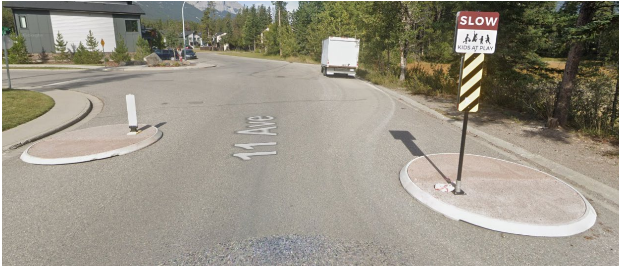
Figure 5: Hawks Bench Prefabricated Traffic Calming Implementation Example
