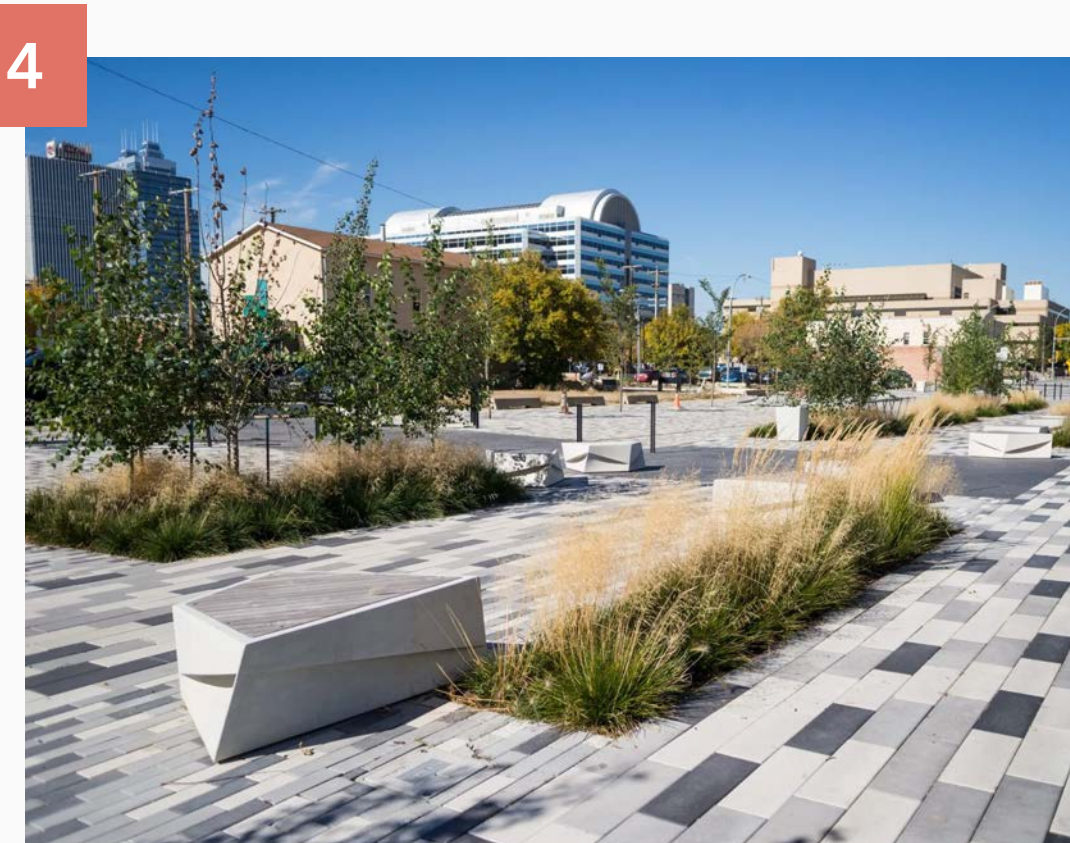
Green stormwater infrastructure can add greenery into streets and public spaces while also capturing and treating stormwater runoff.
