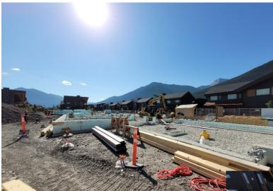
Construction of the south building foundation continues. Another concrete pour has completed the foundation walls for this building. Backfill of the foundation is finished and wood framing can now begin.
