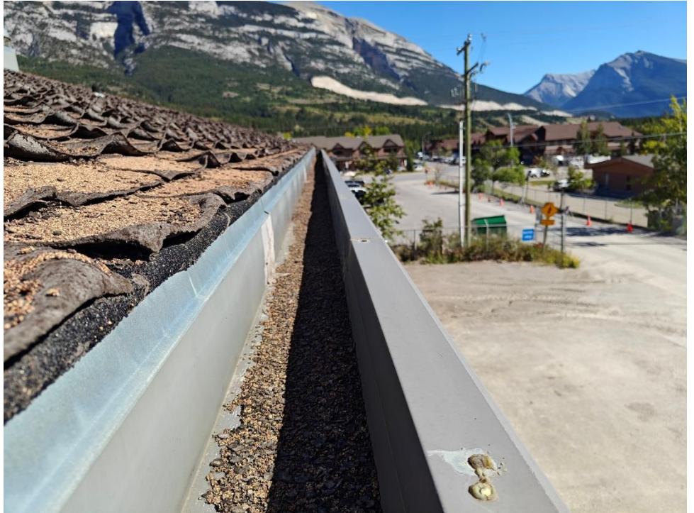
7) Overview of the south gutter and flashing
