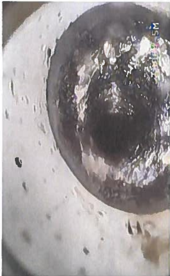
End of PVC at 4.6 m
