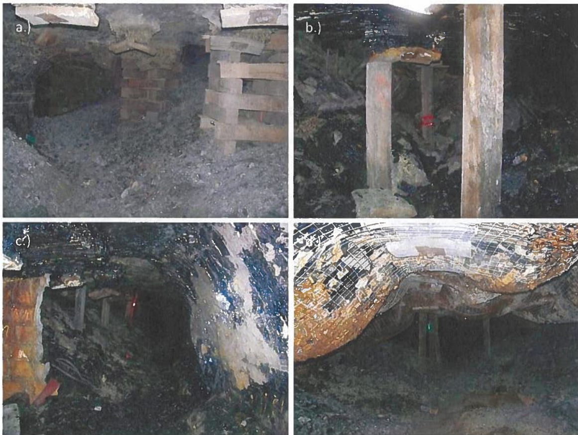
Figure B9. Examples of underground closure in a Pennsylvania longwall coal mine
