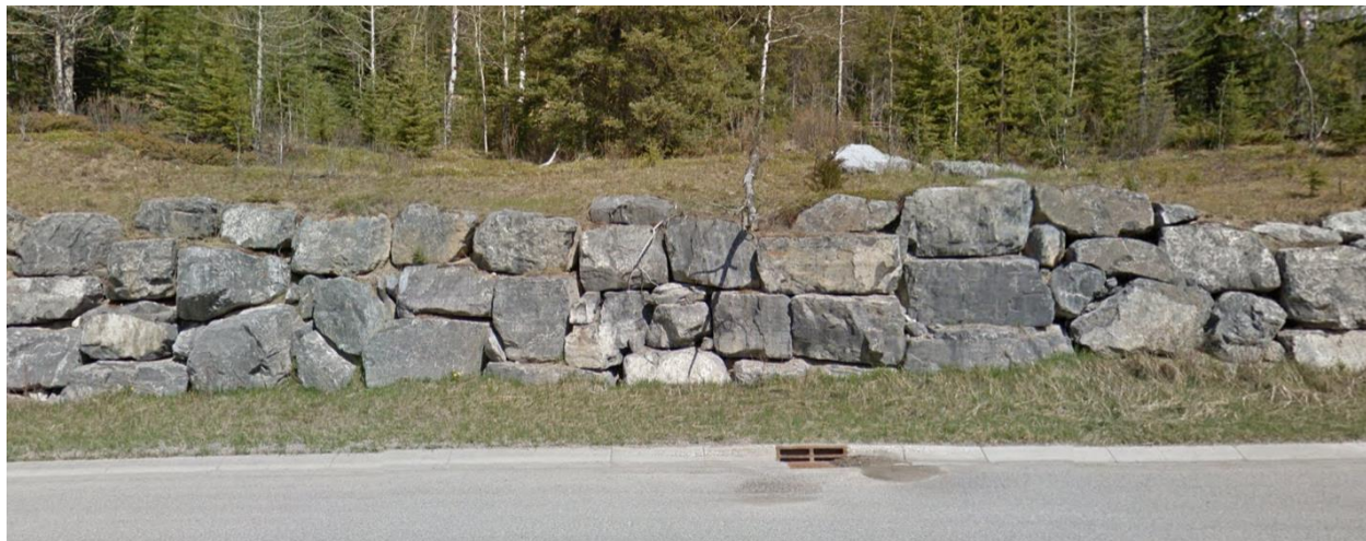
Figure 9-2: Stone Retaining Wall on Silvertip Road, Canmore AB
