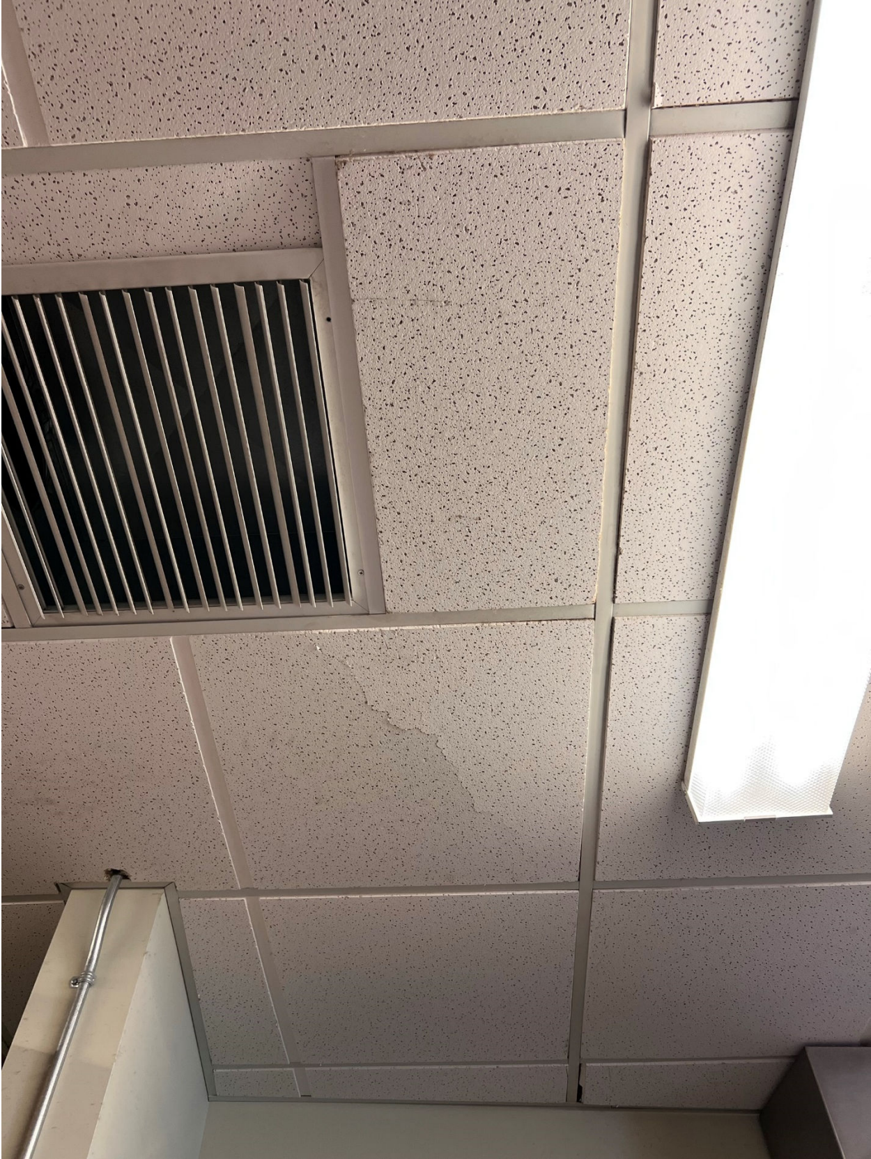
Acoustic Ceiling Panels to be replaced with waterproof kitchen panels
