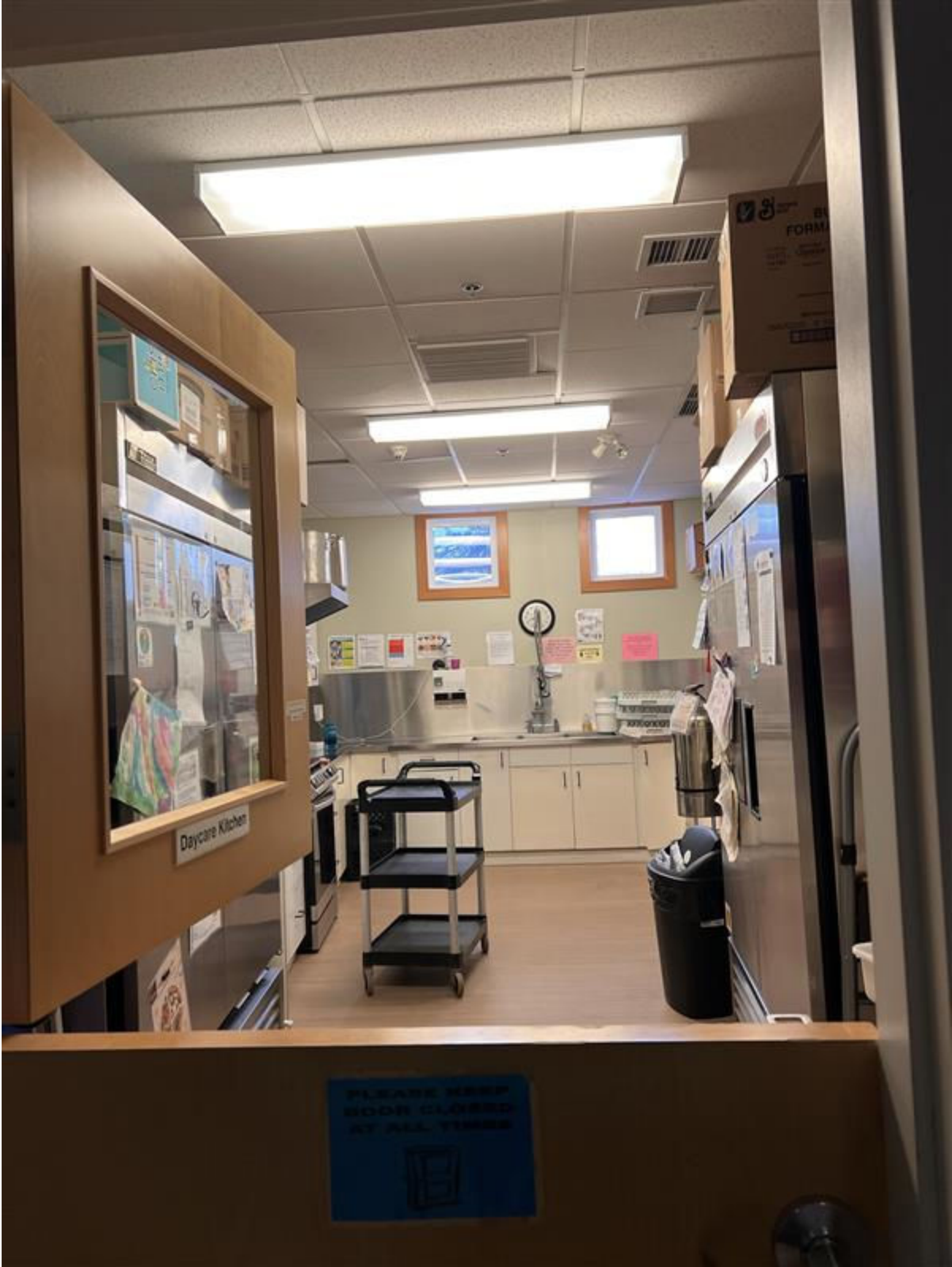
Roundhouse kitchen space. Photos are taken counterclockwise. Door will not be replaced. Door threshold to sink = 22'6".
