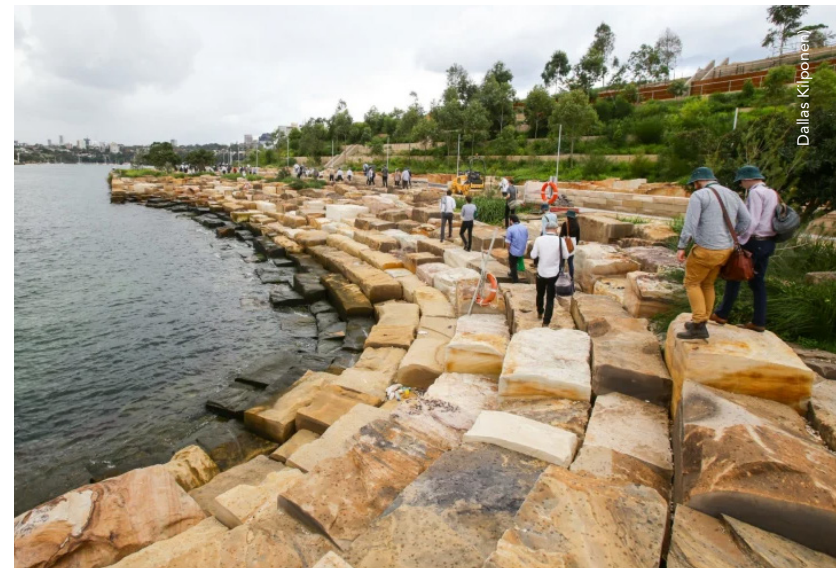
Example of terraced features that can provide seating and respond to changing water levels.
