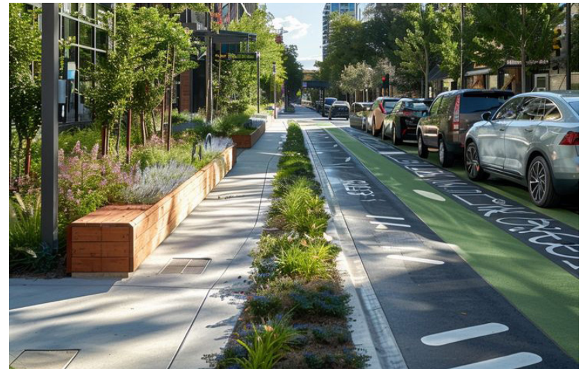
Example of LID infrastructure installed within street cross sections to manage stormwater runoff.
