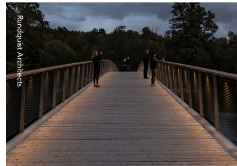
Site-specific, dark sky lighting along a pedestrian crossing
